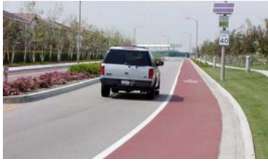
Enhanced streetscape design. Photo Credit: Beckett & Raeder, Inc., Benjamin Tallerico
