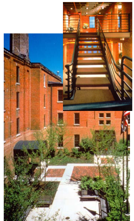
Adaptive Reuse: Argus Office Building (former Argus Camera Factory), and Beckett & Raeder Offices. Photo Credit: CDI
