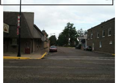
Lack of pedestrian amenities.
